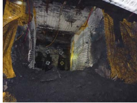
Figure 18: Holing longwall 11 PDRR
