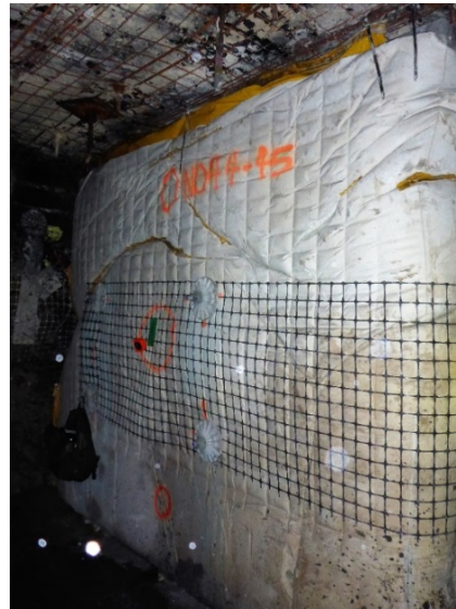
Figure 14: Longwall 11 PDRR grout pillar with plastic sheeting removed – 40 m to hole
