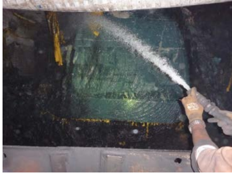
Figure 17: Holing longwall 11 PDRR
