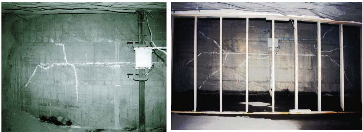
Figure 3 - Formation of yield lines in Meshblock™ seals
