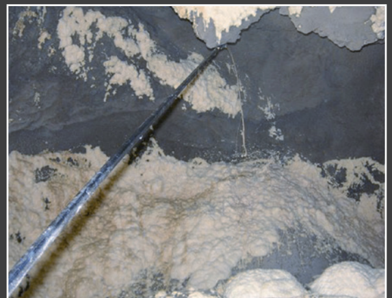
Filling a cavity with Geofoam®
