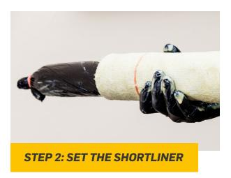
The fibreglass mat saturated with CarboLith PL is wrapped around an inflatable "packer". Ensure that adjacent mats overlap.
