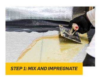
Approx. 2% to 4% of the C-component is added to the A-component, depending on temperature, and mixed thoroughly. The next step is to further mix with a double volume of B-component for a minimum of 2 minutes. A prepared fibreglass mat is then saturated with the mixture using a spatula to both sides of the mat. Finally, a metal roller is used to ensure complete saturation of the mat.
