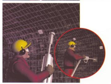
Lower drill and move to next installation. Tool works equally well on wall installations, hold-ing plate, allowing for easy installation.
