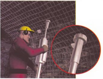
Place magnetic Saab installation tool into the chuck of the drill.
