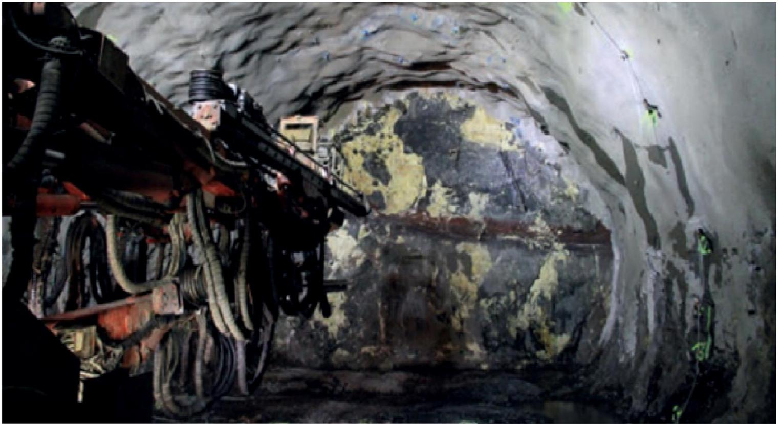
The injection sealing made use of Carbopur WX and accelerators, while at extreme cases at the location, Carbopur WF and additives were injected.
