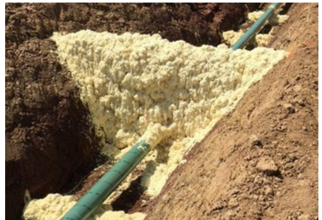
Installed Breaker and Pillows for gas pipeline
