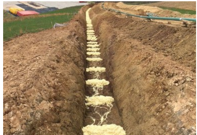
Installed Pillows ready for gas pipeline
